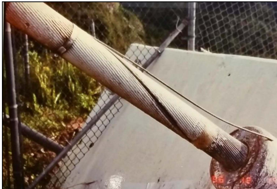
Figure 20: Single wire break observed at ground end of cable B4-1 on 12/12/1996 (photo: NAIC Arecibo Observatory, a facility of the NSF).
