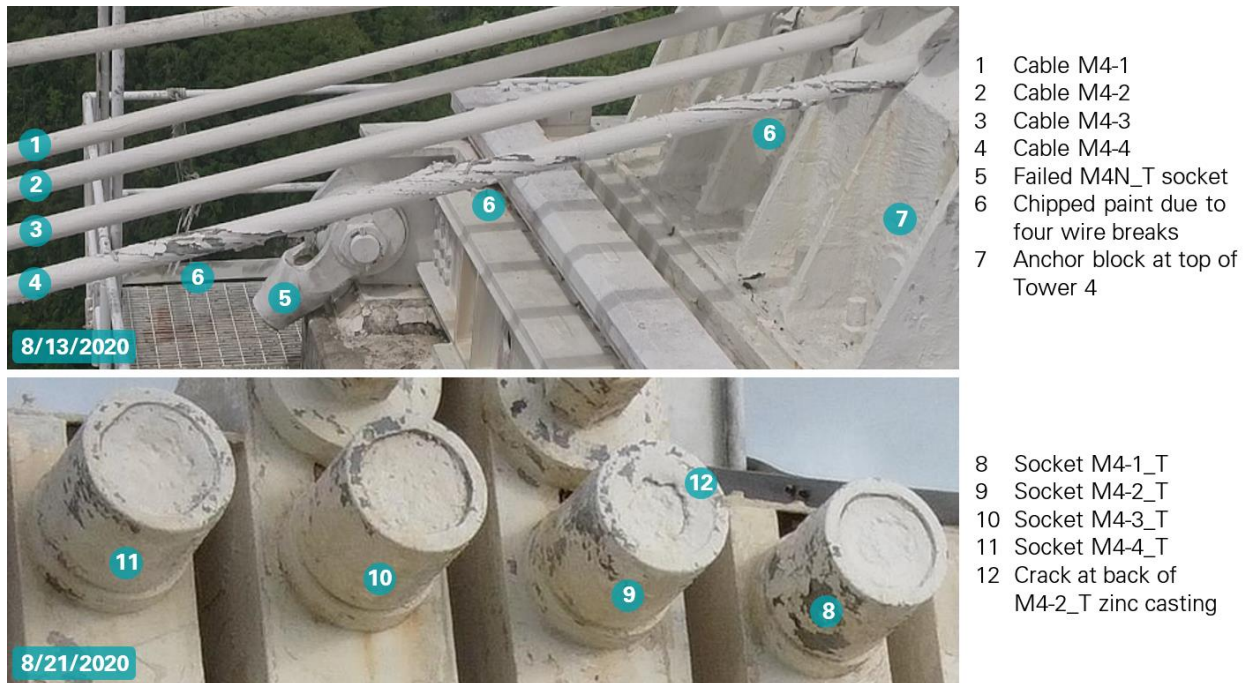
Figure 26: Damage on original M4 cables at top of Tower 4 after first cable failure (photos: NAIC Arecibo Observatory, a facility of the NSF).
