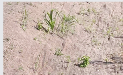
3 Coconut matting for site stabilization
