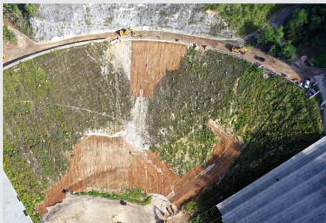
2 Rim wall repairs and erosion control measures
